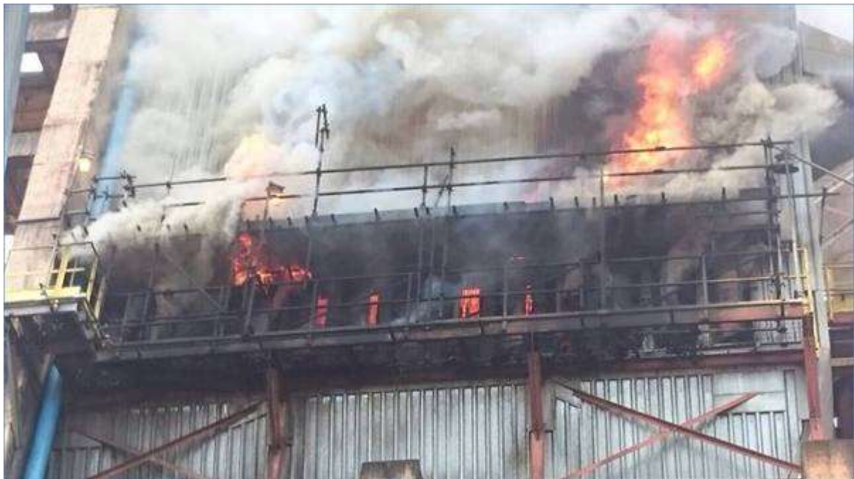
example of successful explosion protection and unsuccessful fire protection
